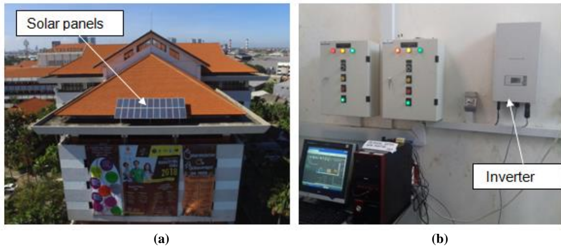
Figure 2. Photograph of the PV system showing solar panels (a) and on-grid inverter (b)
